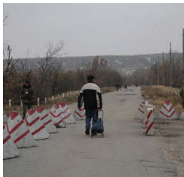
At control point “Stanytsia Luhanska” a man is moving to separatists-controlled Luhansk via the damaged bridge which can be crossed only on foot.
